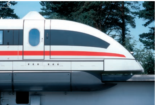
Transrapid unit on maglev guideway
