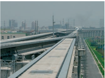
Transrapid vehicle approaching points in the curved position
